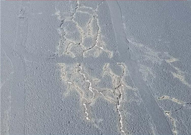
White coloring may also be seen in the cracks or white staining on the surface due to salts. These salts are from winter deicers resulting from excessive use of salt on parking lots during the winter months or from natural earth salts coming to the surface known as efflorescence.
